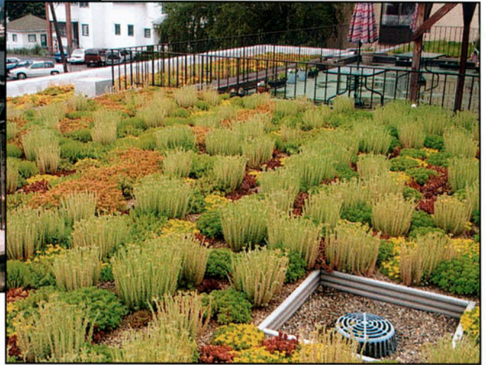
LEFT, SOLAR PANELS. BELOW, ECO-FRIENDLY GREEN ROOFING.
